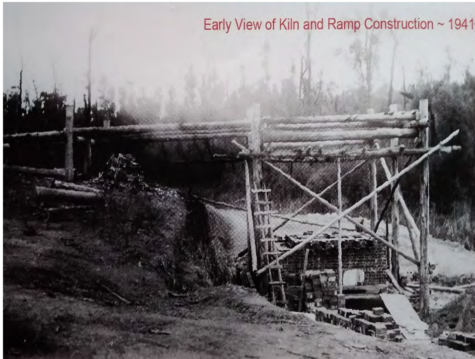
Figure 14. Photo of the process of construction of the kiln in 1941 showing the access ramp to the left and the forest behind which was burnt during the 1939 bush fires. Source: Kurth Kiln 2018 Calendar.
