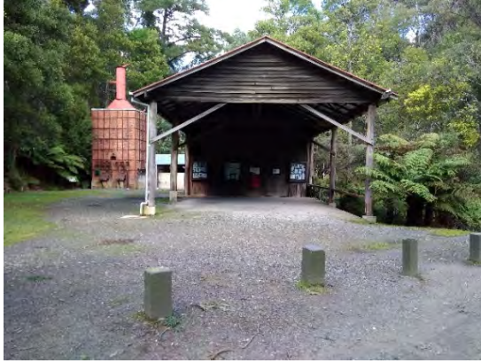
Figure 8. Photo of the large storage shed and kiln taken from Soldiers Road, 2018. Photographer Jane Morton Colbert.
