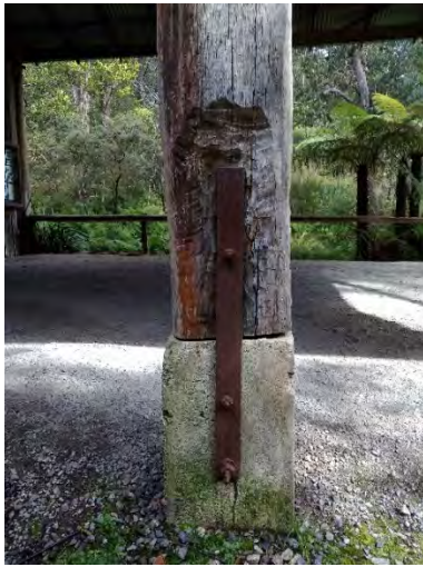
Figure 9. Photo of one of the shed posts strapped to a concrete block, 2018. Photographer Jane Morton Colbert.
