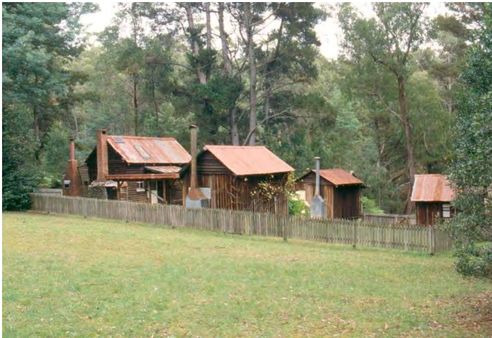
Figure 11. Photo of Kurth Kiln huts sited uphill from the kiln site. Source: Heritage Council Victoria.
