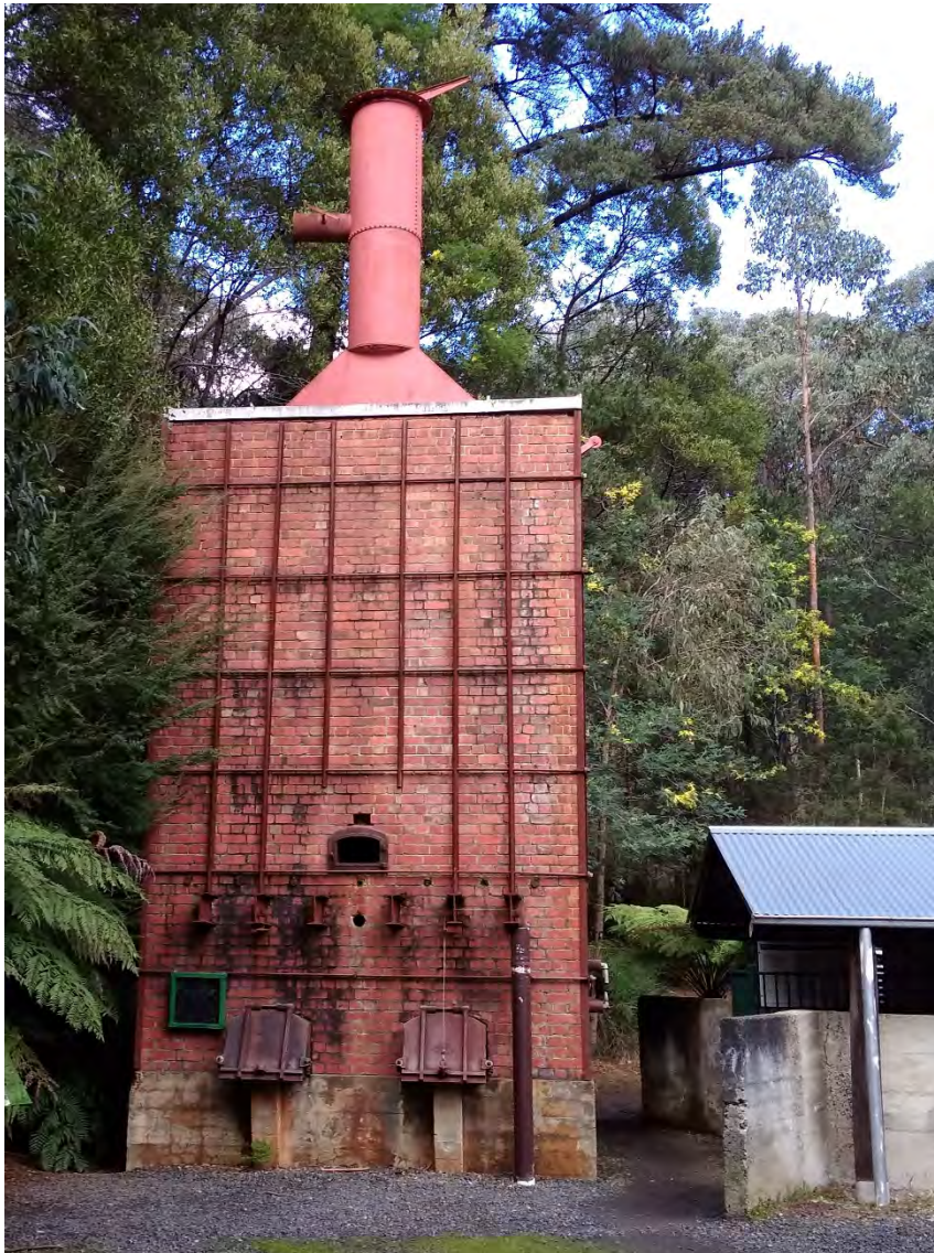
Figure 6. Photo of Kurth Kiln with the blacksmith's forge structure to the right, 2018. Photographer, Jane Morton Colbert.
